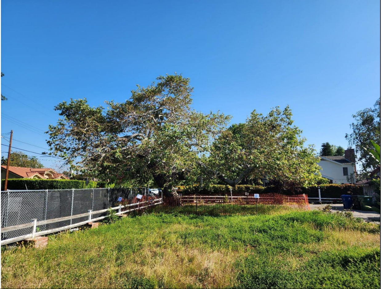
Protective root zone fencing installed.
