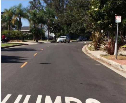
Image for Note 6: The speed hump at the top of this image is visible from the “HUMPS” marking at approximately 200 feet away
